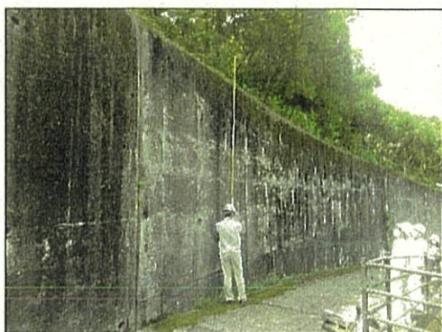
(擁壁の点検の様子)
