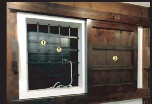
2 nd Floor: Shuttered Window
