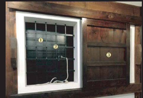
2 nd Floor: Shuttered Window
